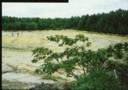
Construction of the production facility.
